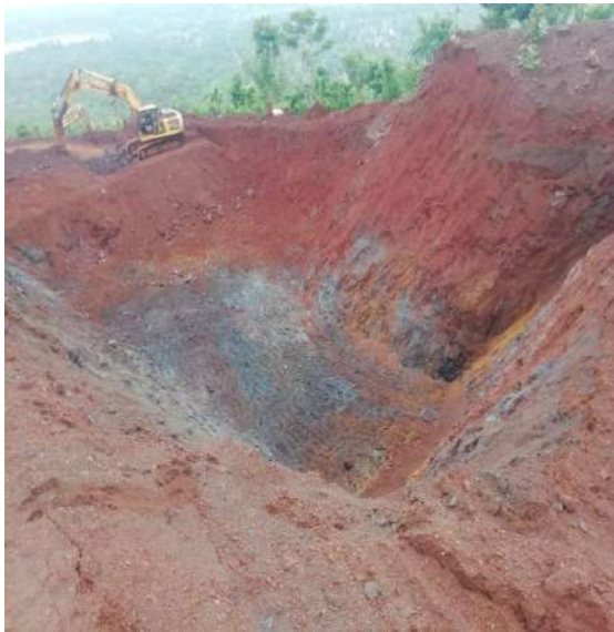
Construction of check dam
