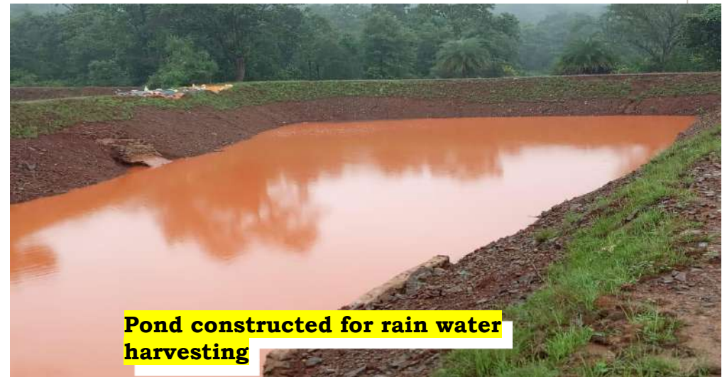
Pond constructed for rain water harvesting
